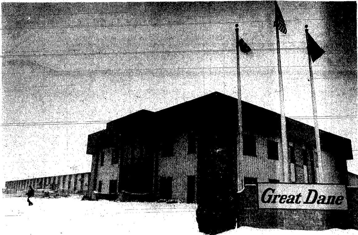
Great Dane truck trailer manufacturing plant in Wayne has been such a growth success that it has paid off low interest loans used in the development of the plant, early. The early pay-back gives the city more than $500,000 in a revolving loan fund that can be used to help other businesses locate and expand in Wayne.
